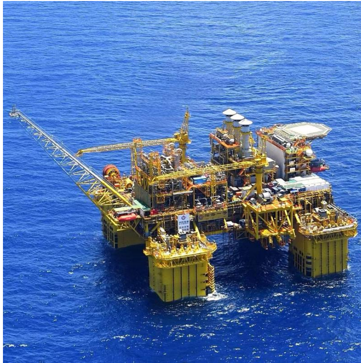
(a) Prediction of heave motion for semi-submersible platforms: semi-submersible platforms are semi-submerged floating structures commonly used in offshore oil and gas exploration, marine construction, and scientific research. Accurate prediction of this motion is crucial for ensuring safe and smooth operations in dynamic sea conditions.
